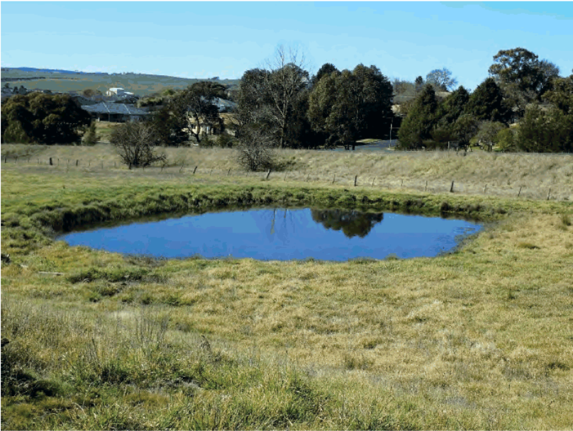
Figure 22 Basin 7A is the lower of the two dams in this location
